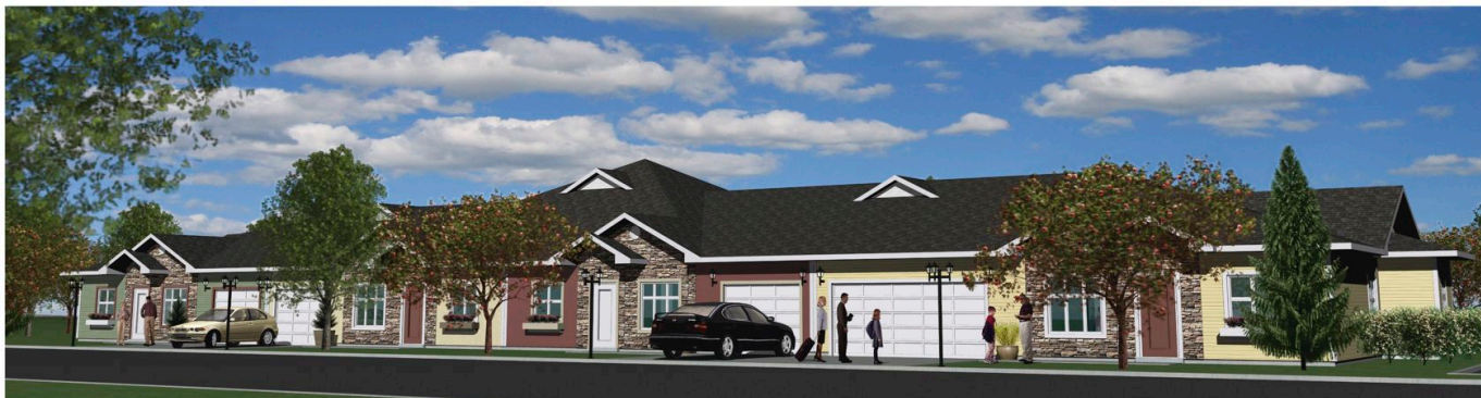
building 1 view from east
